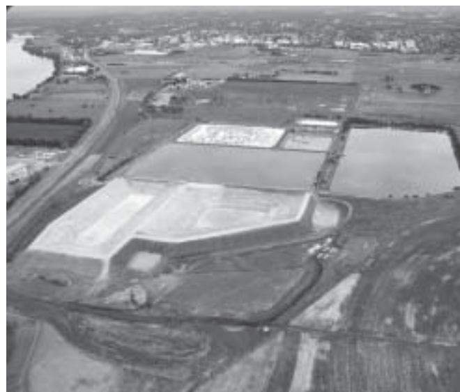
Wet weather storage pond currently under construction
