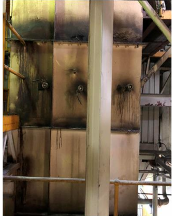
EPA ID 10 – No. 3 Gluten Dryer Baghouse
