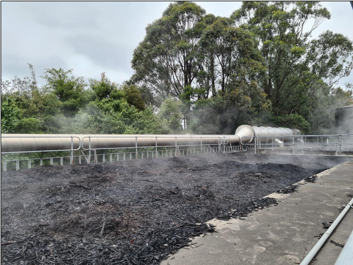
Photo 1 – A view of DDG Biofilter 1 as found on 9 December 2021
