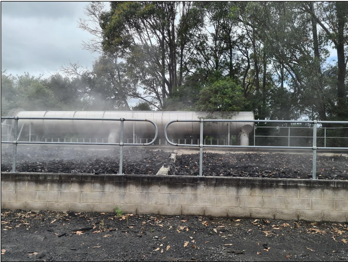
Photo 2 – A view of DDG Biofilter 2 as found on 9 December 2021
