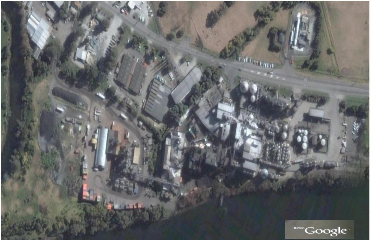
Figure A 1 Shoalhaven Site Aerial Photograph
