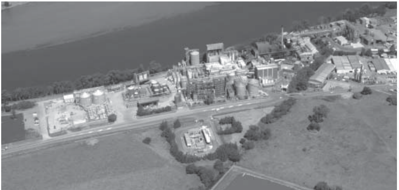
The proposed project will see odours significantly reduced and up to 4.5 million litres of water reused every day
