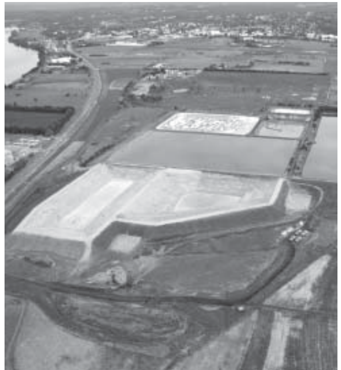
Wet weather storage pond currently under construction
